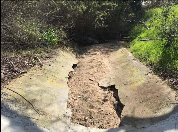
Representative Photograph 3. Facing NW. Portions of concrete is broken and in need of repairs.
